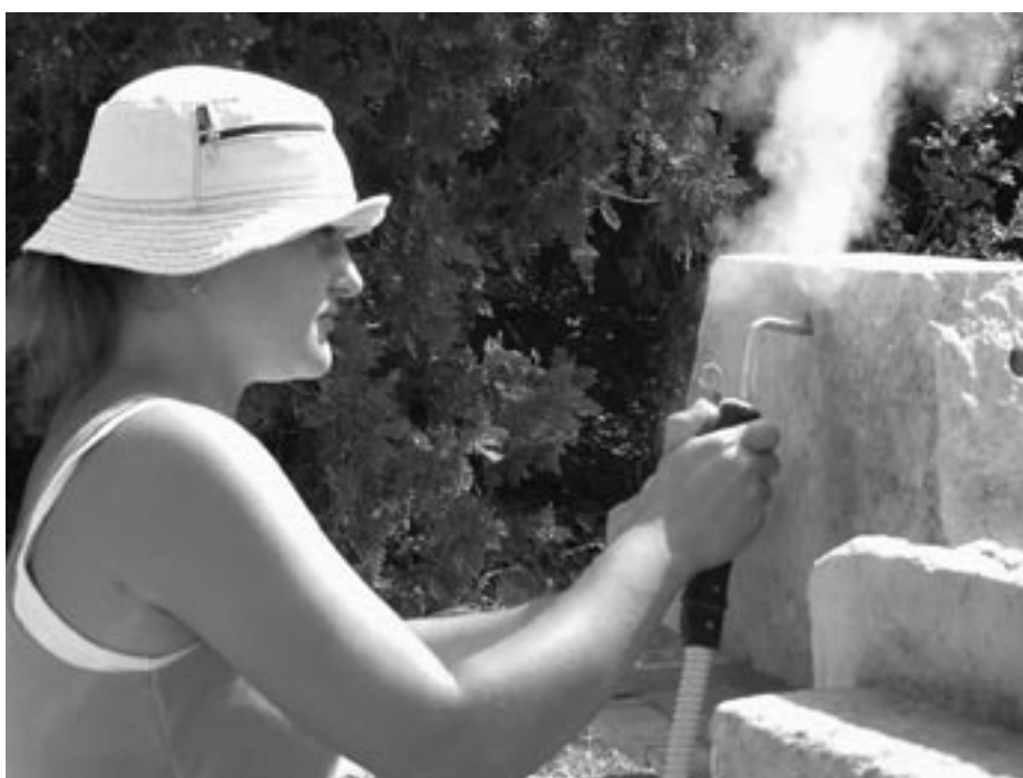
Figure 1. Botanical colonization is removed from a monument fragment by steam cleaning.
