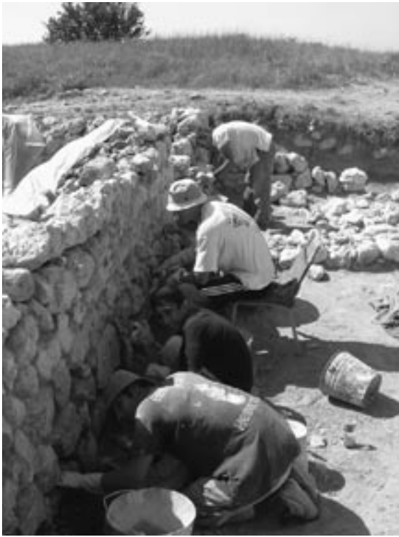
Figure 2. Pointing team applies mortar to an ancient structure at Chersonesos.
