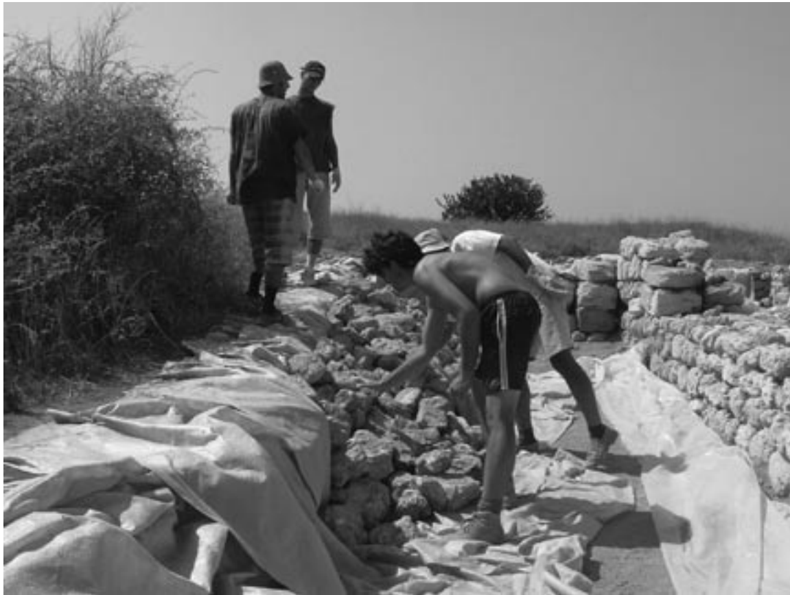
Figure 4. Team members build a temporary rubble retaining wall to stabilize an earthen bank.
