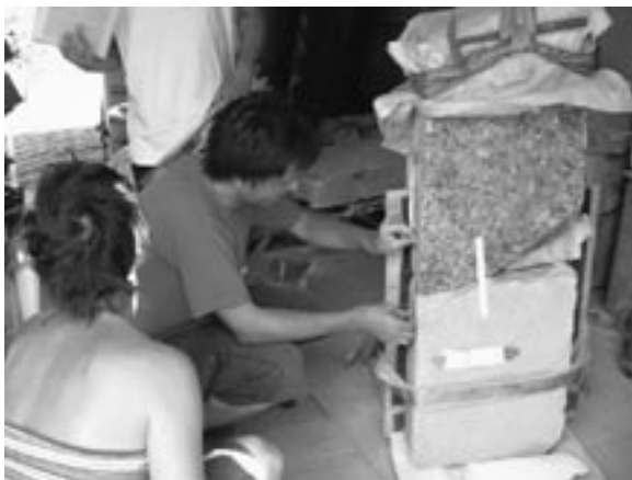
Figure 3. Points for locating reinforcing rods are determined.
