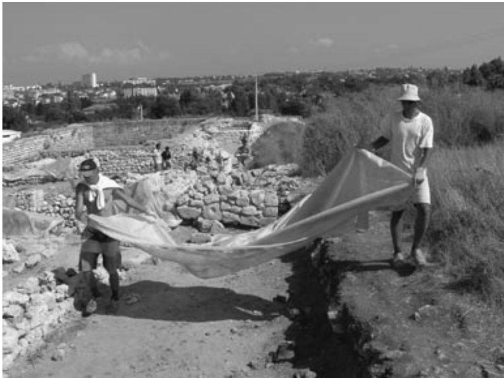
Figure 3. Laying geotextile to control plant colonization.
