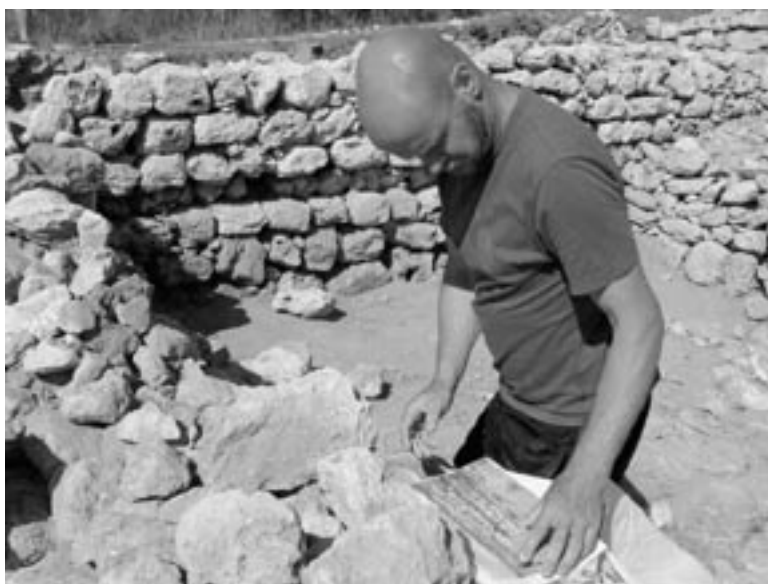
Figure 2. Jonathan Kemp refers to a detailed wall-face photograph to help reconstruct a section of collapsed wall.
